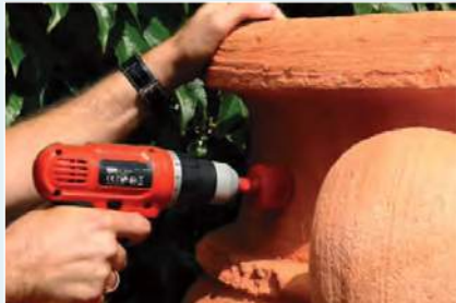
A hole is drilled in the tank for the installation of the inlet seal.
