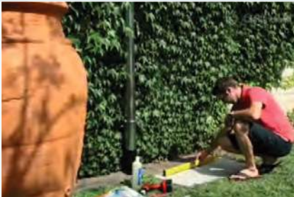
The ground must be level for the installation of a tank.
